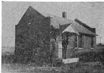
The transmitter building of WTRC, Elkhart, Ind. DXer Roger Mais, who submitted the picture, is standing in the doorway.
